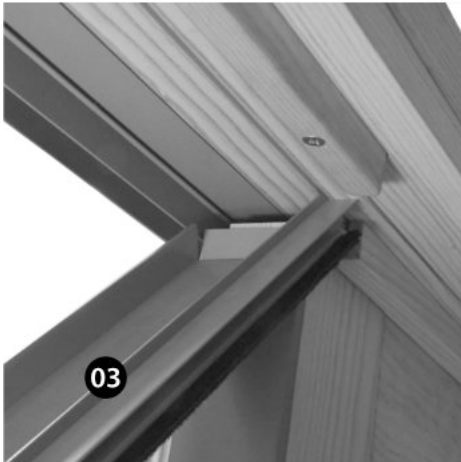
Align Exterior Head Stop in Head Jamb
