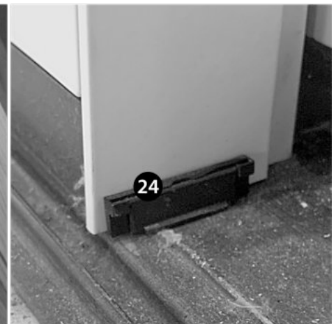
Install Weep Cover(s)
