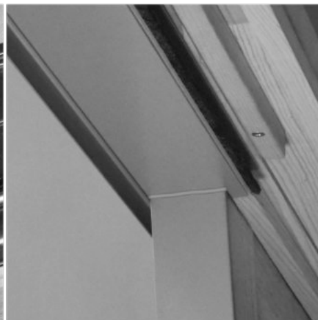
Apply Sealant To Head Seam
