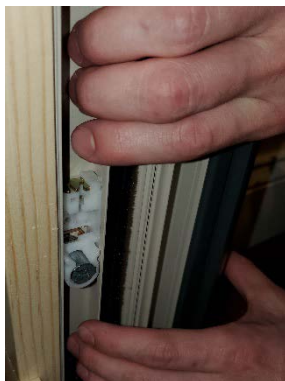
Flex jambliner center away from the balance shoe
