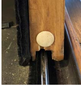
Figure 1: Circular Cap in place
