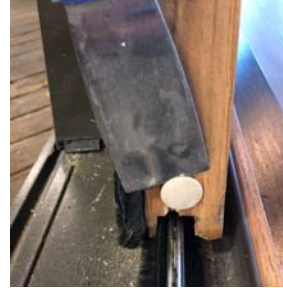
Figure 2: Putty knife removing circular cap
