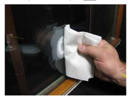
4. If after removal of exterior frost/moisture by wiping with IPA and paper towel, there is moisture visible on the airspace side (#3 surface) between the panes of glass the unit is considered failed. If no moisture is visible between the panes of glass the unit is not a failure and should not be replaced.
